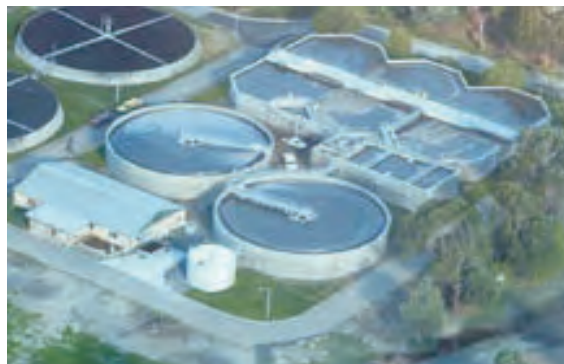
Figure 10.7 An aerial view of a sewage plant
