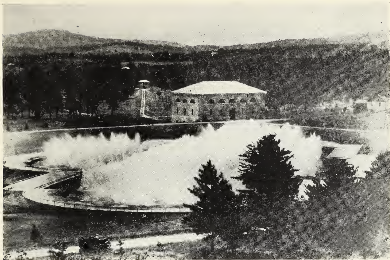
AERATING PLANT AT CROTON, N. Y. Aerating water by spraying it into the air and sunshine helps in killing disease germs, and at the same time gives the water a better taste.
